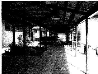
Steel structure & roof
